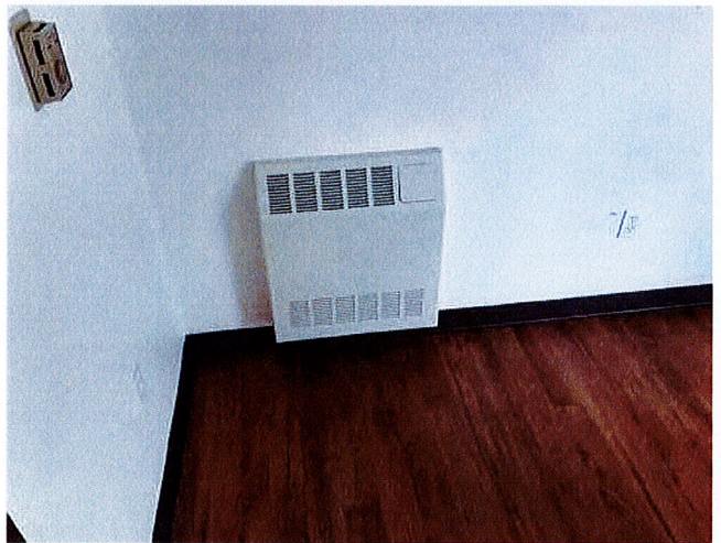
28 - HYDRONIC FAN COIL
