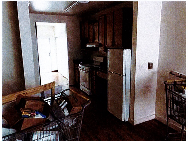
40 - UNIT 206, OCCUPIED, KITCHEN
