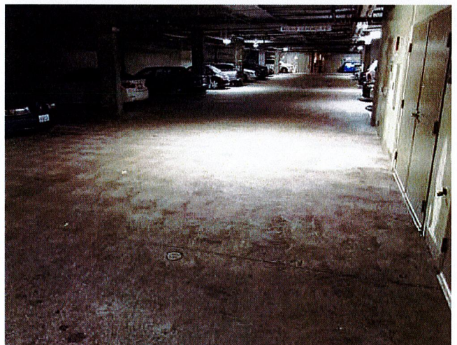
6 - UNDERNEATH PARKING AREA
