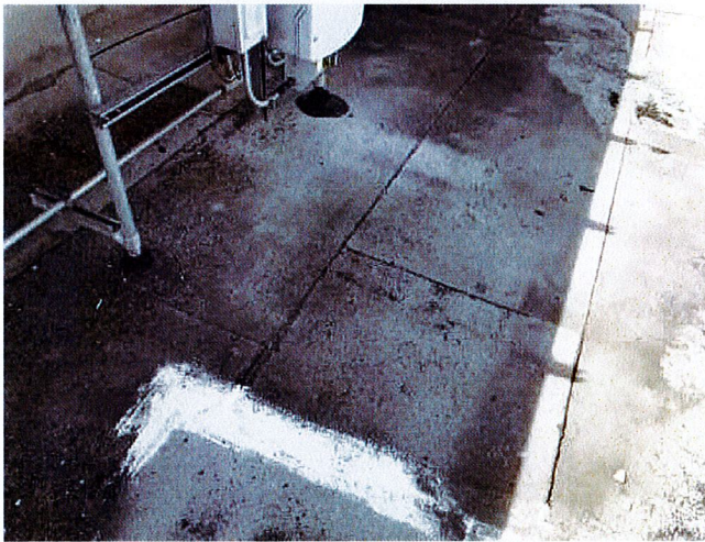
15 - MODIFIED BITUMEN ROOFING
