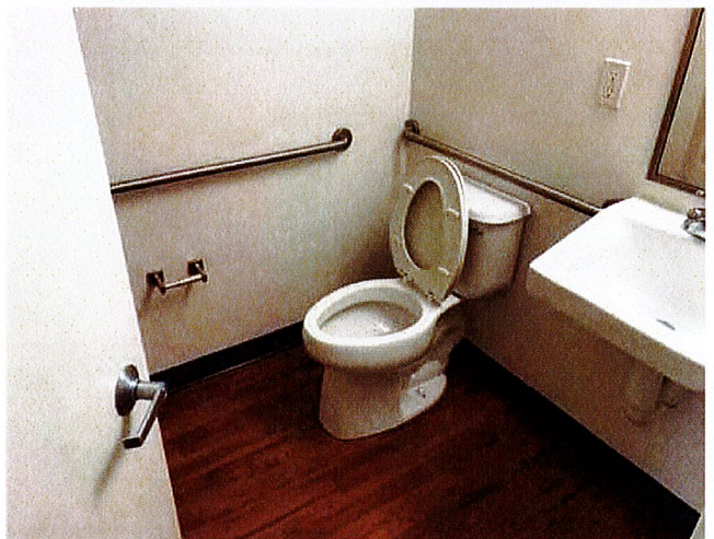
36 - UNIT 206 , VACANT, BATHROOM
